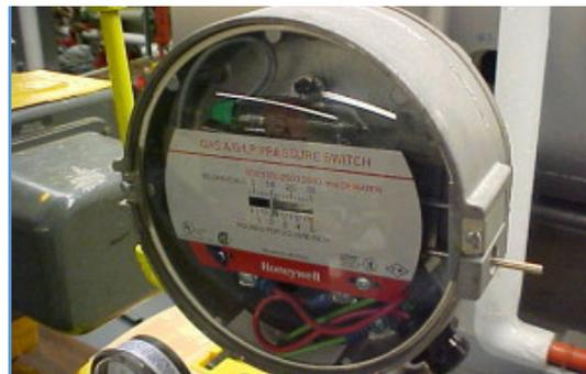
In our opinion, the installation of these kinds of test valves only meets the intent of 8.2.8 when they are installed to make for an interlock by having both switches (high and low gas pressure) taken off from the same sensing line.
