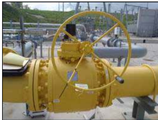
Figure 2-3 Trunion Mounted Style Ball Valve with Gear Wheel Operator and Position Indicator
