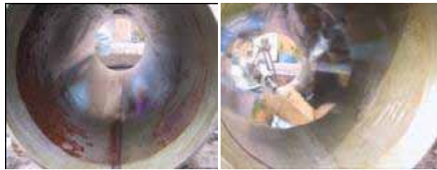
Figure 4-2 Inside of Pipe Before and After Water Jet Flush
