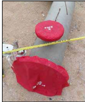
Figure 4-3 Foreign Material Exclusion Covers on Pipe Ends
