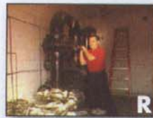
PHOTOS Q, R, S, T, and U. Leaking plug valves.
