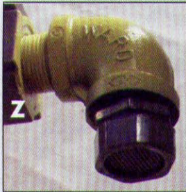
PHOTOS X, Y, and Z. Vent Terminations can be blocked with insect nests.
