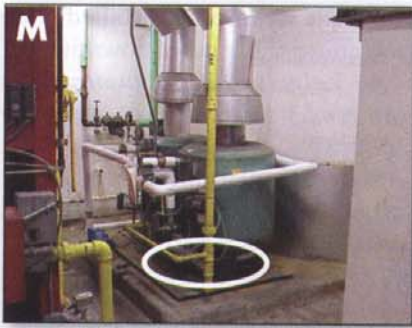
PHOTO M. Flame roll-out (hard starting) can be a warning for dangerous conditions that may get worse.
