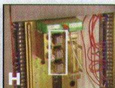
Photos G and H. Obsolete burner management systems.
