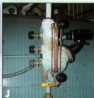
PHOTOS I and J. Valves in the instrument lines can render switches / instruments ineffective.
