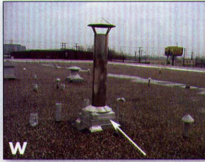
PHOTO V (Typical gas-train vent valve) and W (Typical vent termination on roof).
