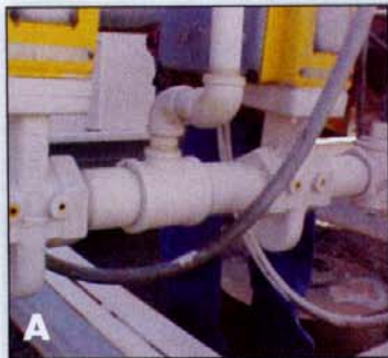
PHOTOS A & B. Tightness testing of safety shut-off valves and blocking valves is not being carried out.
