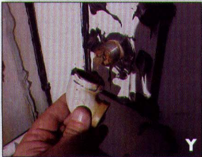
PHOTOS X, Y, and Z. Vent Terminations can be blocked with insect nests.
