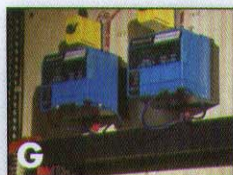
Photos G and H. Obsolete burner management systems.
